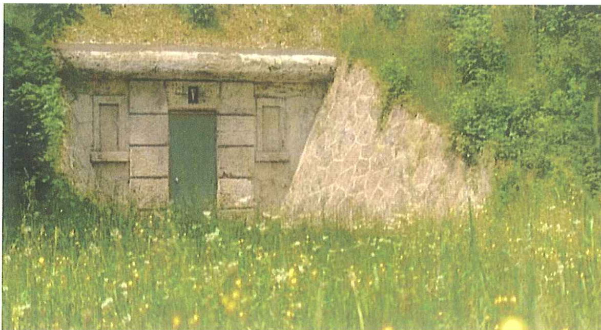
captage (source SWM)
